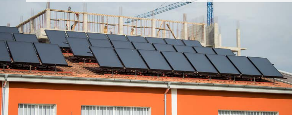
The Orthopedics Clinic of the main hospital in Pristina is one of the first 32 public clinics and schools that have been upgraded with energy efficiency and renewable energy investments as part of the WBG’s Energy Efficiency and Renewable Energy Project in Kosovo.
